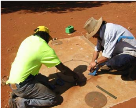
Checking the septic tanks.
