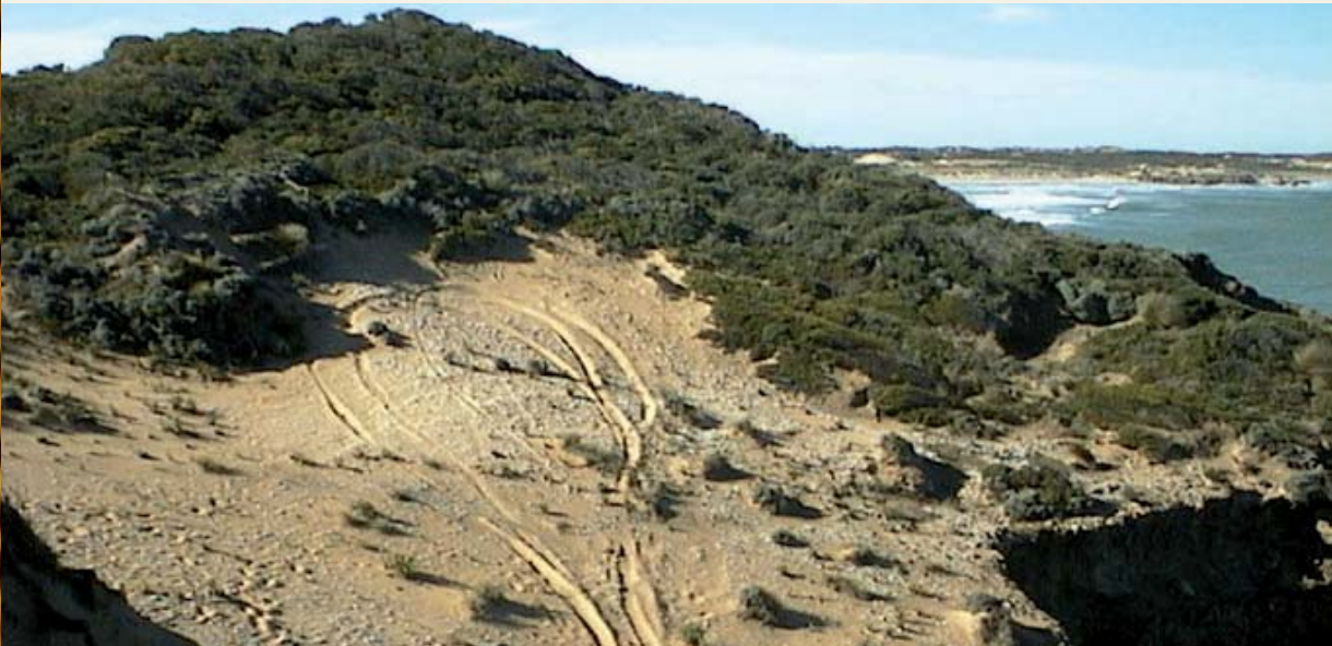
Site damaged by recreational vehicle use, now protected under a conservation plan [Supplied by Aboriginal Heritage Branch (DPC-AARD)]
